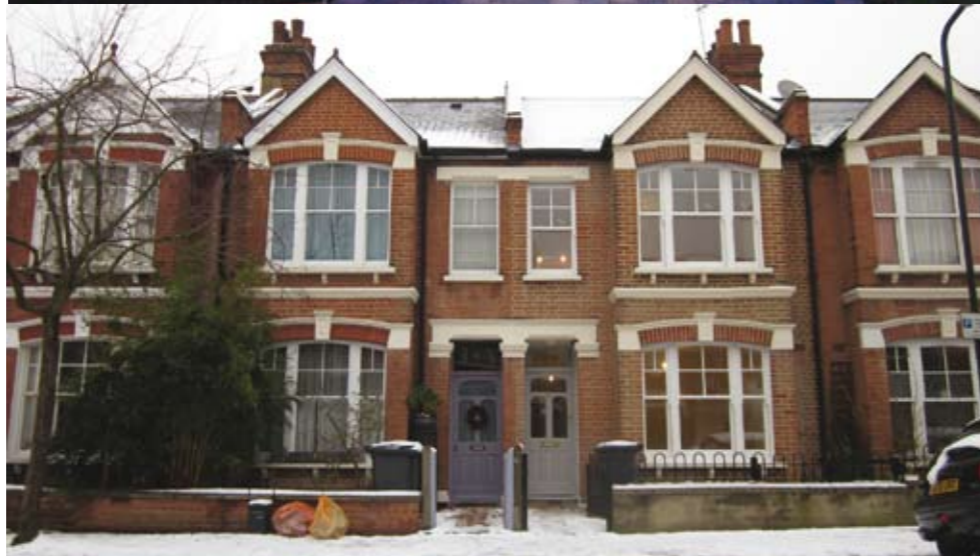
Retrofit for the Future project, Balham (Prewett Bizley Ltd)
